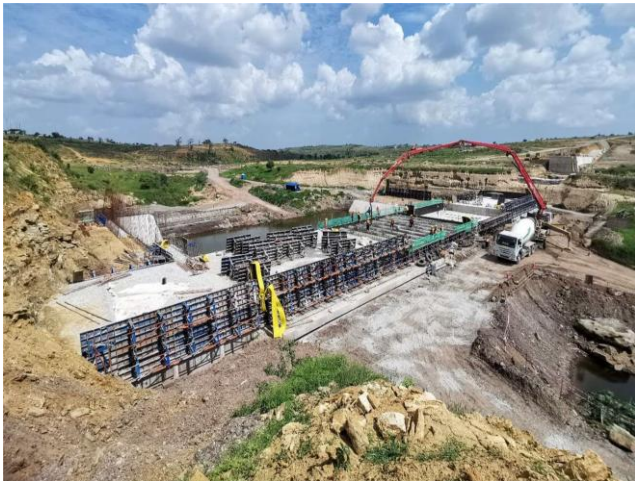
Lower Check Dam: casting concrete surround for the drainpipes
