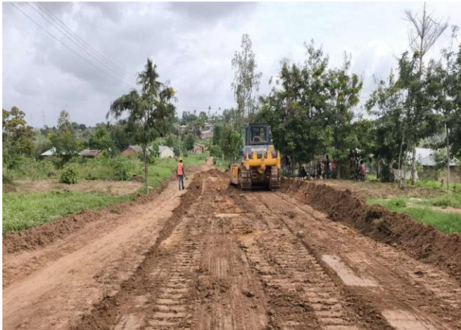
Ongoing site clearance and topsoil stripping: Road B, Ch. 3+500
