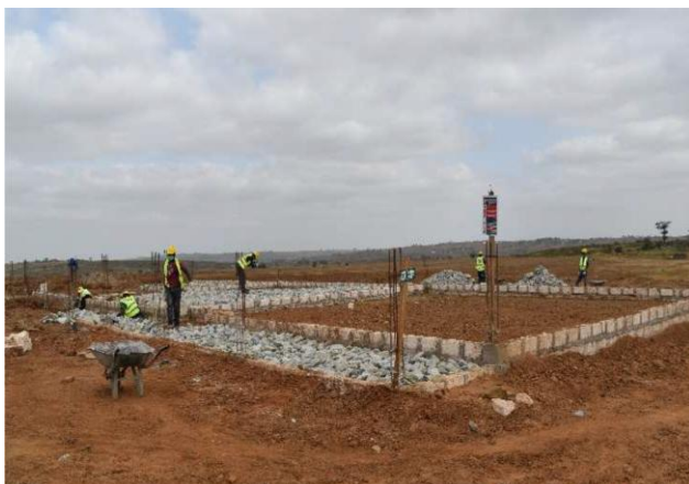
Nunguni Primary School: Blinding concrete placing for classrooms
