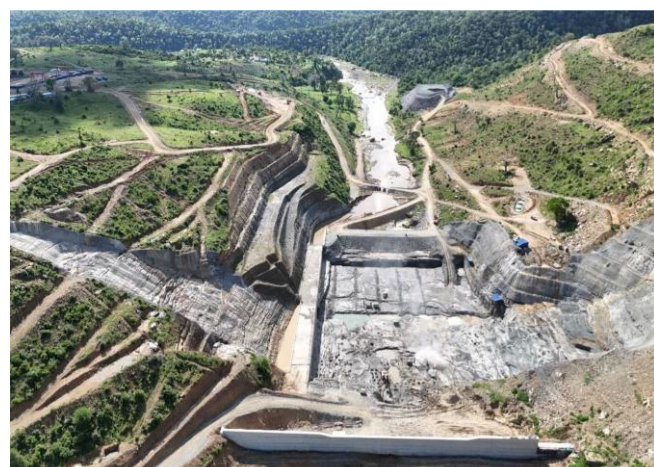
Main Dam: Excavation and Slope Protection Completed
