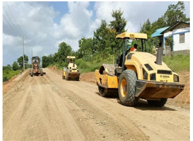
Ongoing processing and compaction of subgrade layer: Road A, Ch. 0+780
