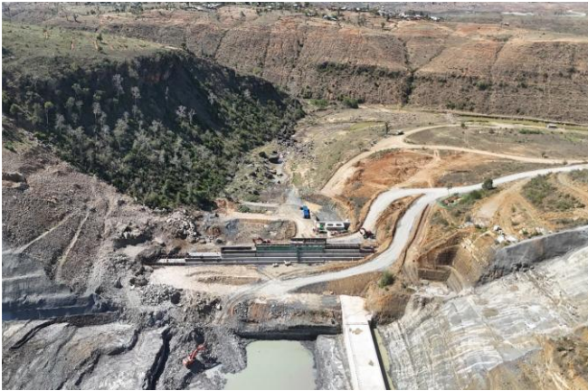
Main Dam: Excavation and Slope Protection Completed
