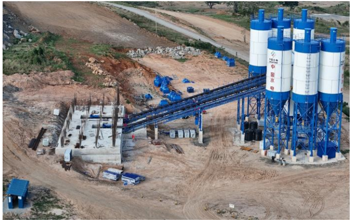
Installation of the third batching plant at Main Dam
