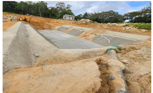
Kwale County Development Support: Backwash lagoon blinding concrete
