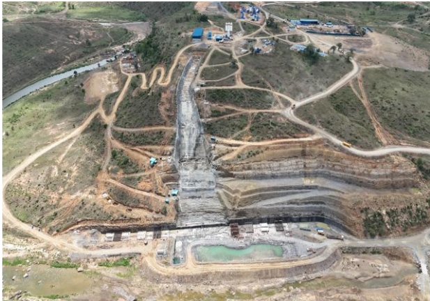
Main Dam Left Abutment: Excavation and Slope Protection Completed
