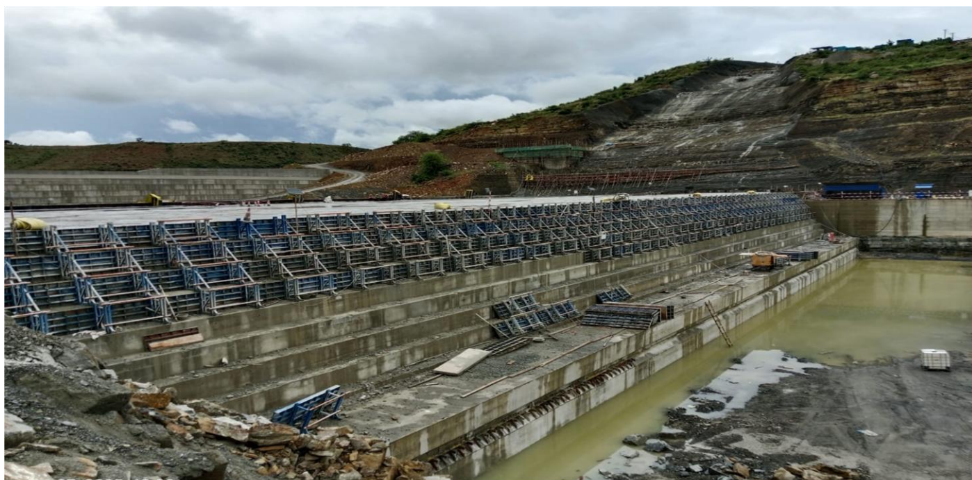
Main Dam: RCC lift 1 completed, from elevation 17.6m to Elevation 28.4m. Height of 10.8 meters of the main dam is already done
