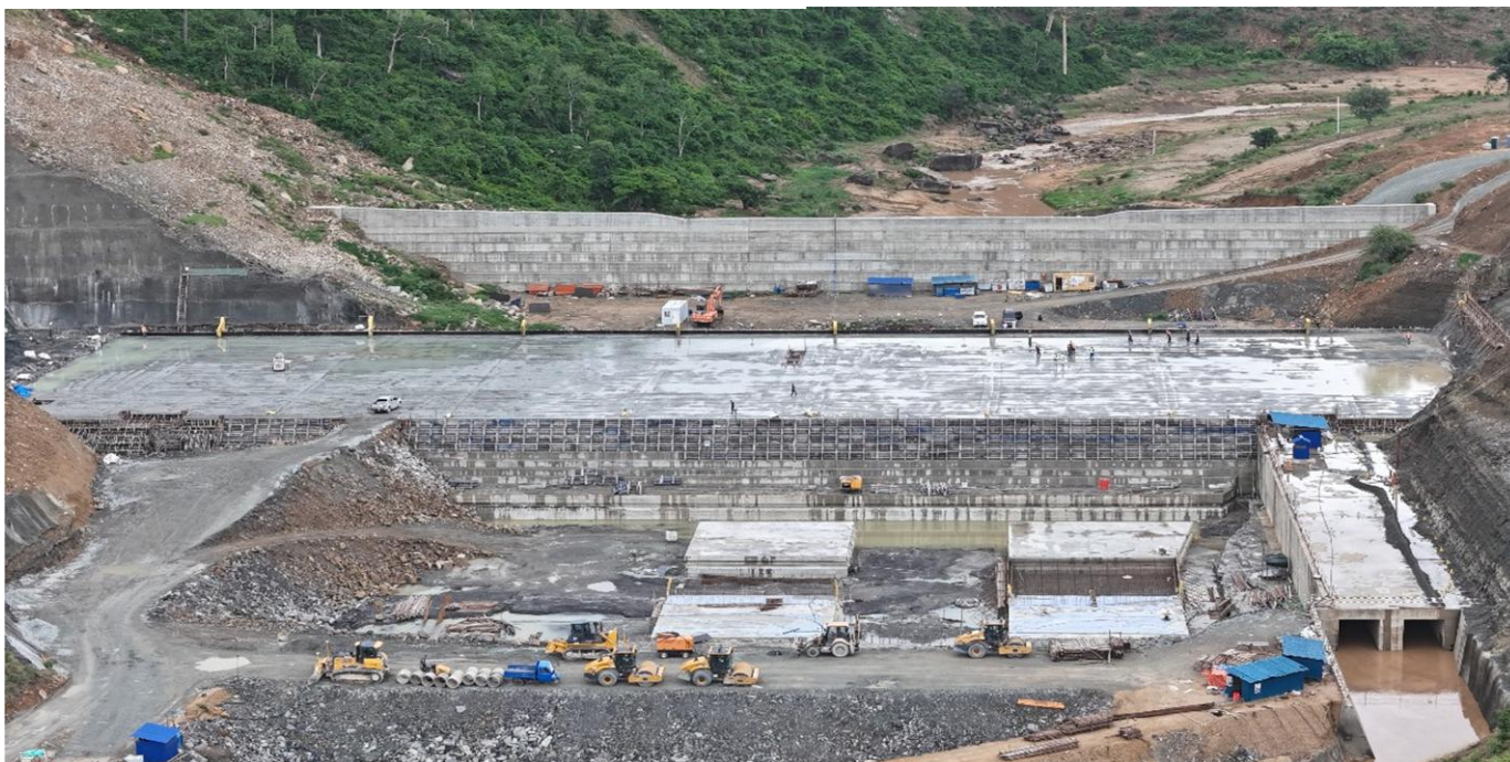
Main Dam: Main dam RCC layer 36, elevation 28.4m as of 27 th April 2025, curing ongoing
