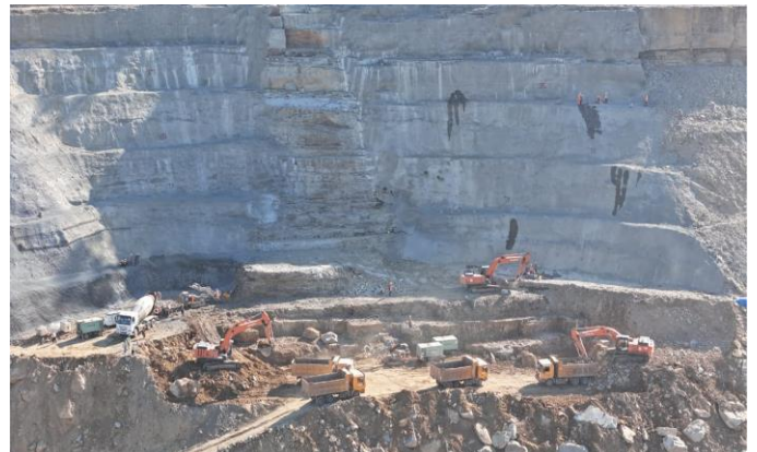
Main Dam Right Abutment: Excavation and Slope Protection Ongoing
