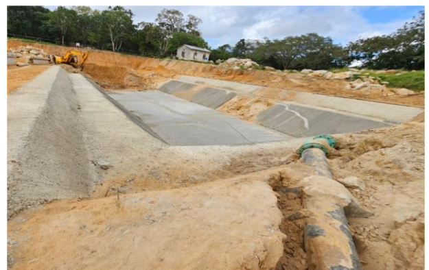
Kwale County Development Support: Backwash lagoon blinding concrete
