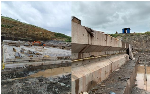
Lower Check Dam: Concrete works at the stilling basin
