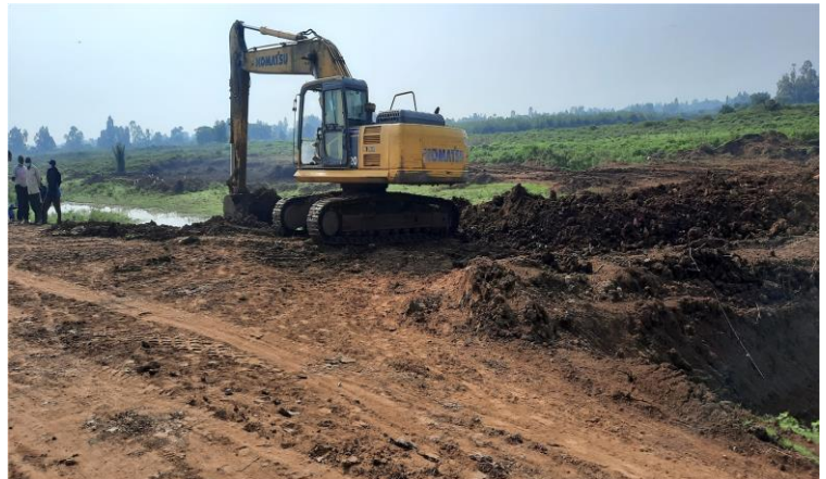
Ongoing construction works for the installation of the sluice gates on the northern dyke to drain floods water to River Nzoia
